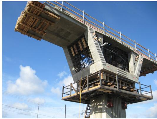
The design for the southwest bridge originally called for a steel tub girder bridge; however, it was redesigned and value engineered to be a precast segmental box girder bridge - **the first precast segmental bridge constructed in WA**. The redesign provided a more economical bridge with extended design life and reduced maintenance.
