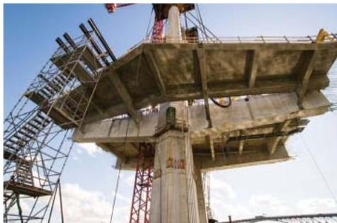
To fill the voids on the underside of the edge girder the contractor chose to use US SPEC STR Mortar, a flowable, shrinkage compensated structural repair mortar with Ferrolok™ Integral Corrosion Inhibitor. STR Mortar solved the problem of making structure repair in hard to reach areas easier and faster for the contractor.
