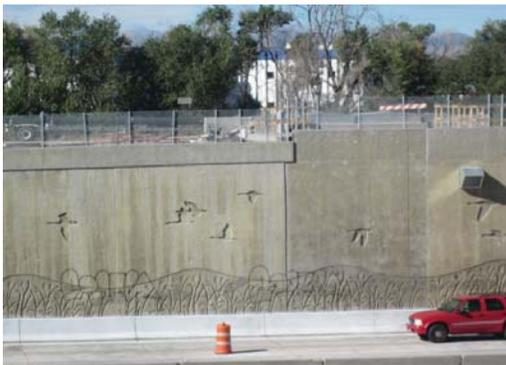
*Yellowing of concrete curing and sealing compounds can lead to unsightly results*
