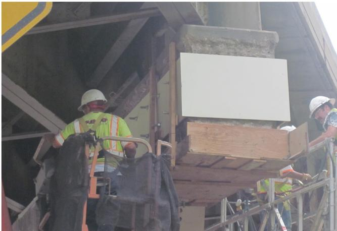
US SPEC STR Mortar, approved by CDOT, was selected for these repairs. STR Mortar was chosen because it is specifically designed for flowable form-and-pour and form-and-pump applications where high strengths are required. With a low water/cement ratio of .34, high fluidity and an extended initial set time, STR Mortar delivered the solution CDOT needed. STR Mortar is a durable repair material achieving 8,000 psi in 24 hours and over 12,000 psi in 28 days.
